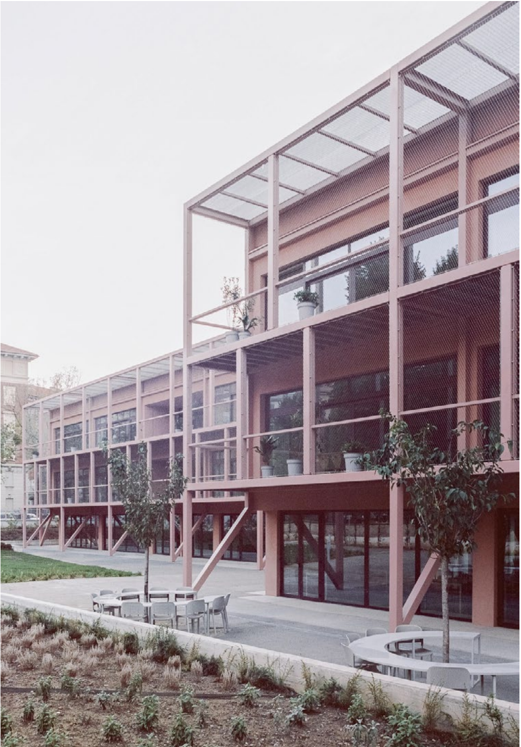
1. View of the addition towards the garden. Ph. Simone Bossi Fermi School (2018).
