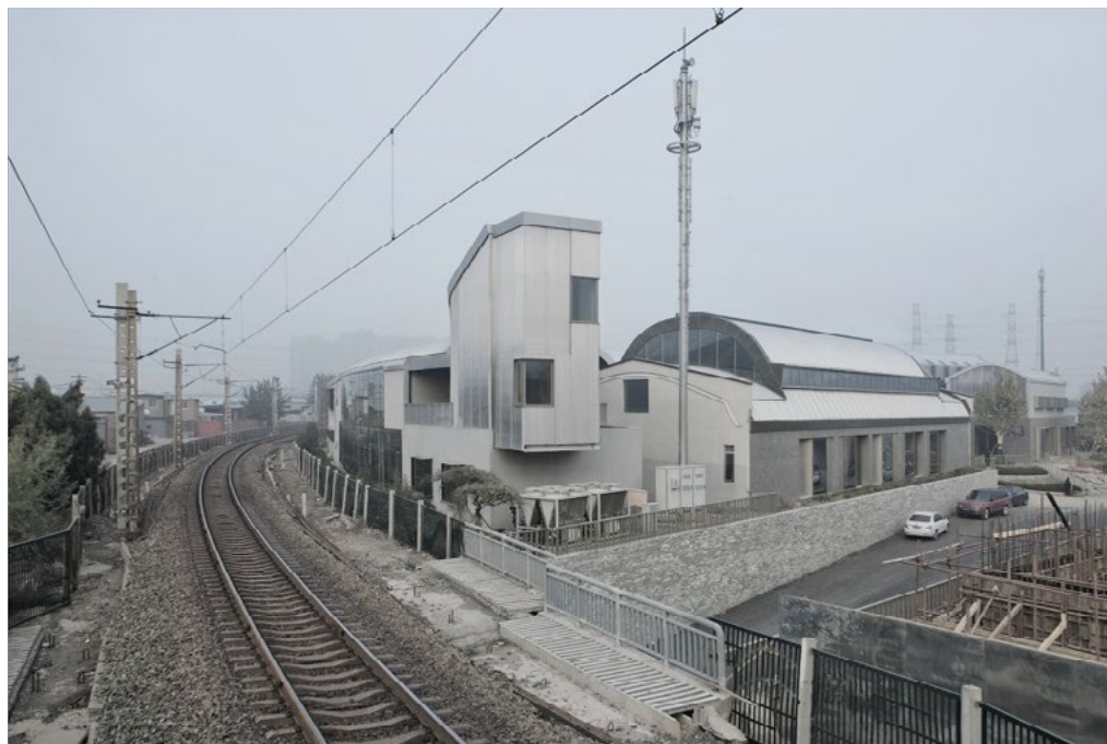
5: Atelier Liu Yuyang Architects, Beijing Cidi Memo iTown, Chaoyang District, Beijing, 2015-2016 [Xia Zhi © Atelier Liu Yuyang Architects, 2016].
