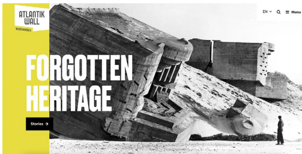
2: Atlantik Wall, Waddengebiet, Danimarca. Home page del sito internet [Atlantik Wall Waddengebiet official web site].
