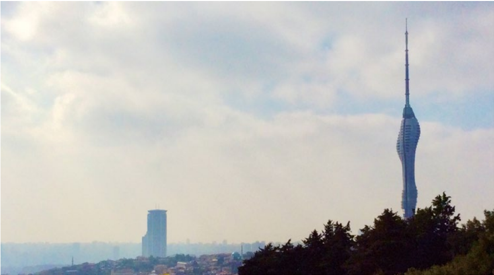
3: The KCTV Tower on the top of the Küçük Çamlıca Hill [Photograph by Luca Orlandi 2019].
