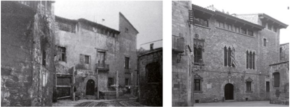
3: The Canon's houses in the Gothic Quarter, before and after the restoration work carried out between 1927 and 1930 by Jeroni Martorell [Photograph by anonymous author; Photograph by Giacomo Alessandro].
